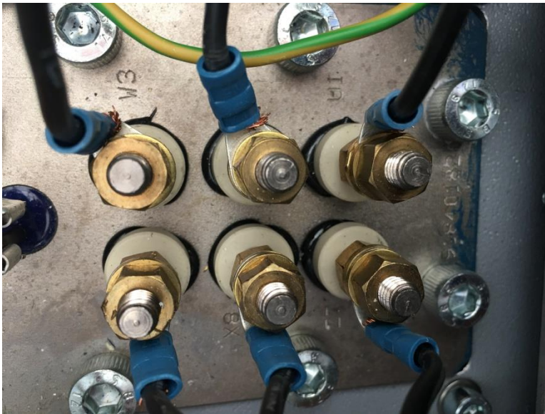
Figure 3: Terminals at the junction plate
